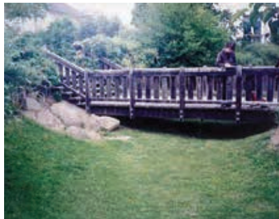
Detention basin, Northhants
