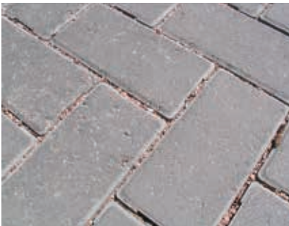
Permeable paving, Cambourne
