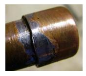
Once soldered, allow to cool naturally. DO NOT wipe with a rag, as this will diturb the solder as it soldifies and could lead to a leak in the future through movement during the cooling process.
